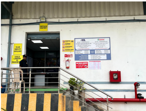
Castrol Warehouse, Bhiwandi
